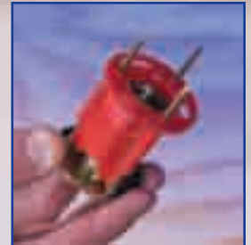
Set Wood-Knocker into place
