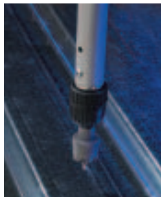
Drill Deck Holes
